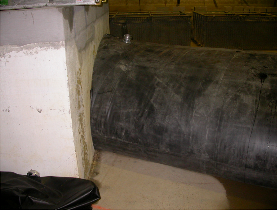
Figure 4. Unit A abutting the wingwall and showing one of the upper fill ports
